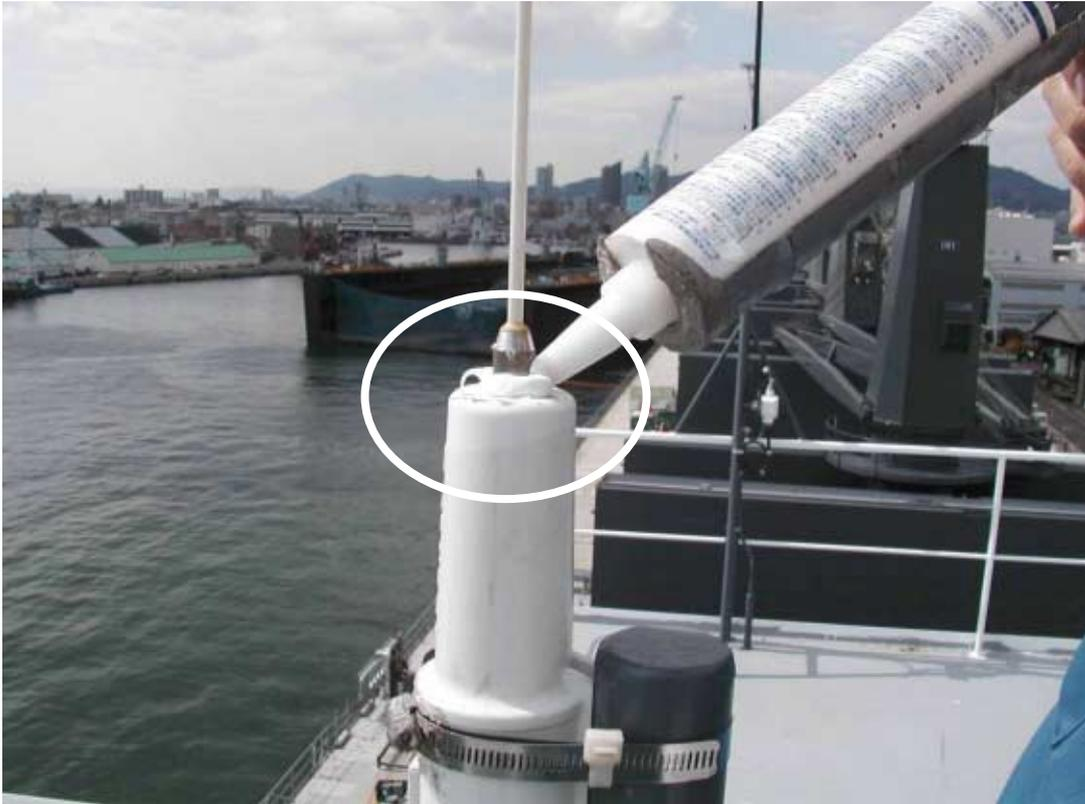
*Fig. 3-16 Waterproofing of whip antenna base*
