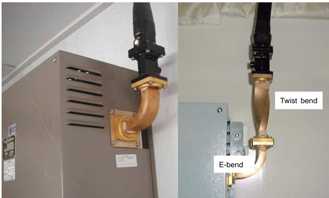
Fig. 1-24 Connecting waveguide to transceiver
