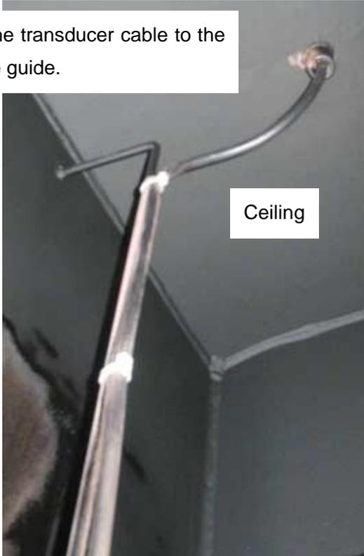
Fix the transducer cable to the cable guide.
