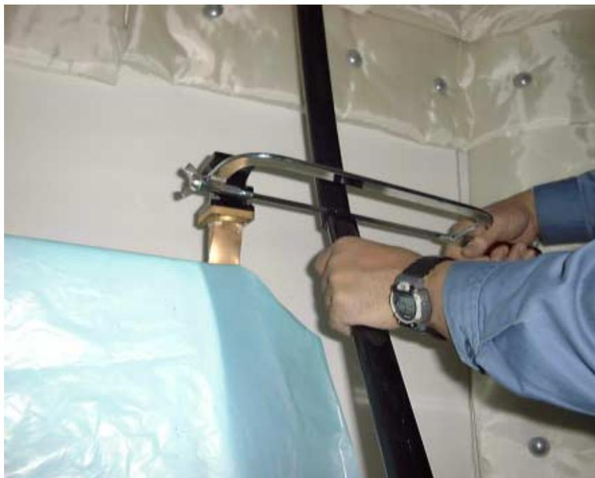
Fig. 1-18 Cutting waveguide
