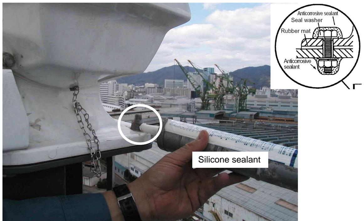
Fig. 1-4 Applying silicone sealant
