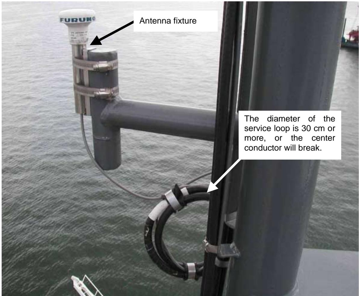
Fig. 4-1 Installing GPS antenna
