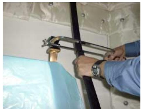
2. Remove the sheath 40 mm using the tubing cutter and scale.
