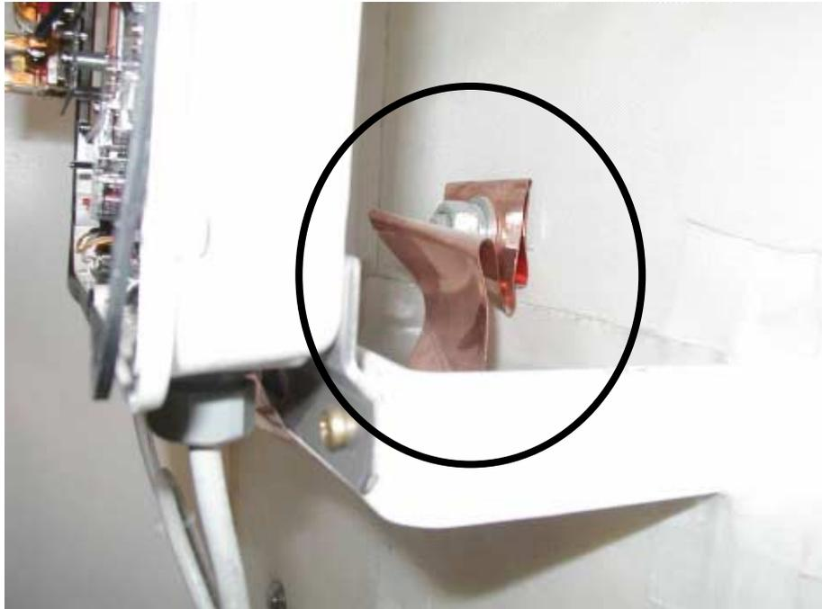
Fig. 3-10 Grounding antenna coupler
