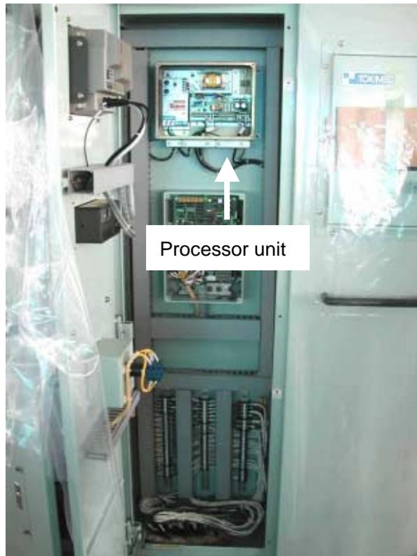
Fig.5-50 Installation of FE-700 processor unit
