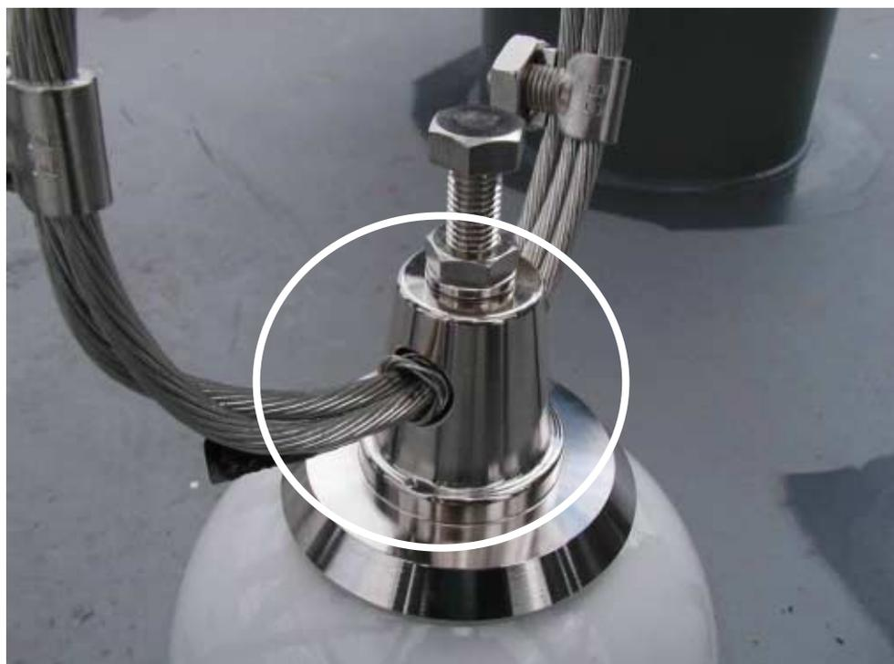
*Fig. 3-6 Fixing antenna wire*
