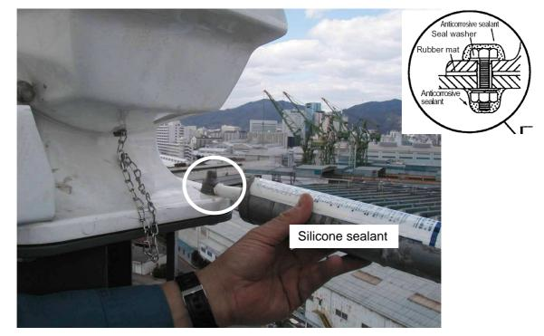
Fig. 1-4 Applying silicone sealant
