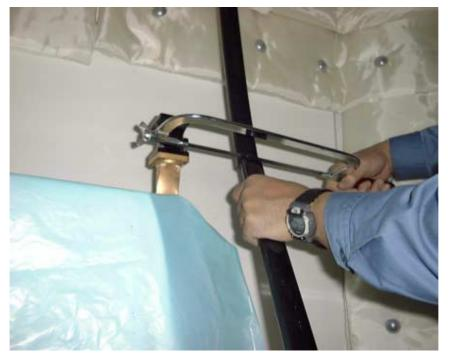
Fig. 1-18 Cutting waveguide
