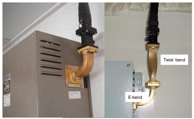
Fig. 1-24 Connecting waveguide to transceiver
