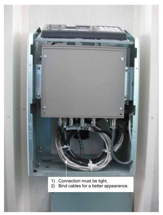
Fig. 3-26 Cables in VHF console
