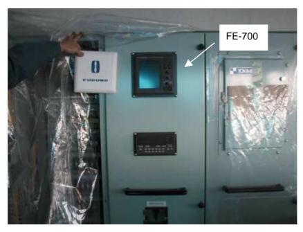
Fig.5-48 Installation of FE-700 echosounder
