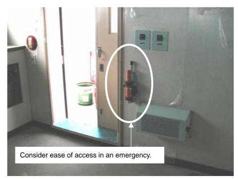
Fig. 3-32 Installing SART
