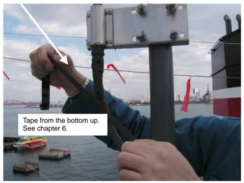
Fig. 3-12 Waterproofing of antenna connector
