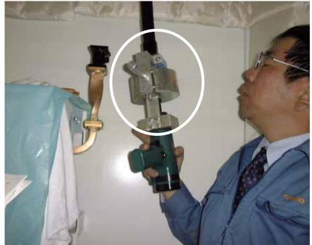
Fig. 1-20 Widening waveguide opening
