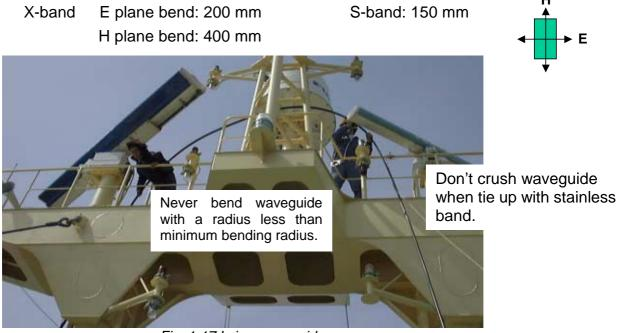
Fig. 1-17 Lying waveguide
