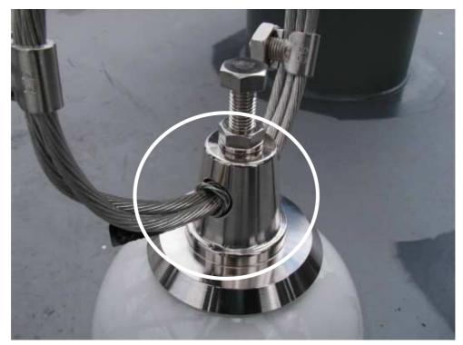
Fig. 3-6 Fixing antenna wire
