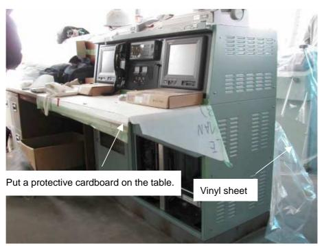
Fig. 3-19 Radio console with protective cardboard
