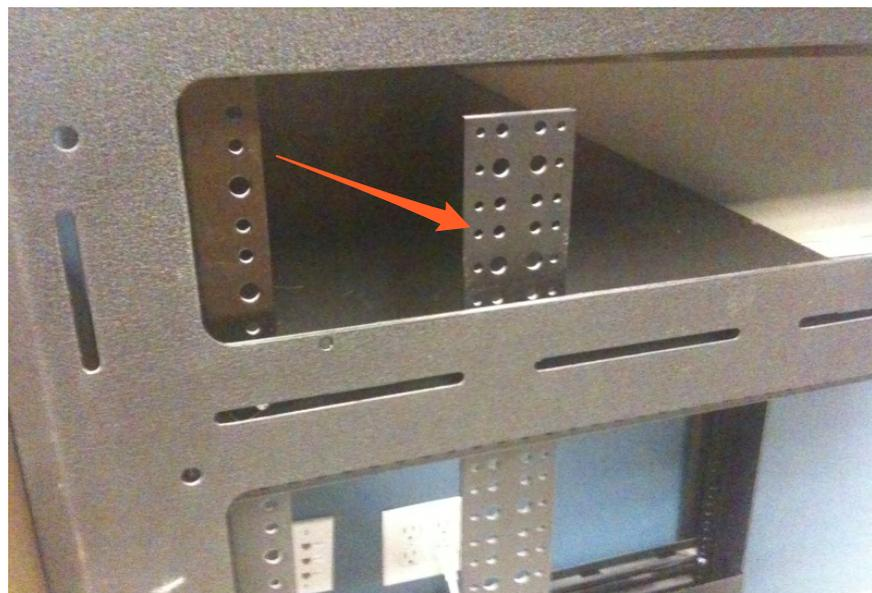
The back and middle mounting points are where you typically want to attach the rack rails to your rack. If you don't have a middle mounting point, then you'll have to use the front mounting point.
